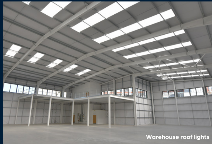
15% warehouse roof lights increasing natural lighting
