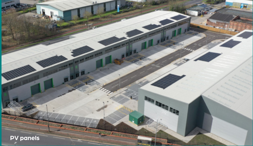
Warehouse roof lights
