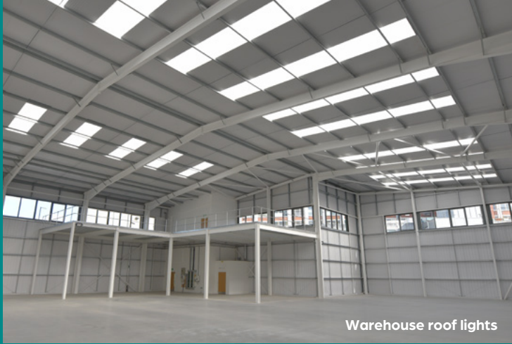
15% warehouse roof lights increasing natural lighting
