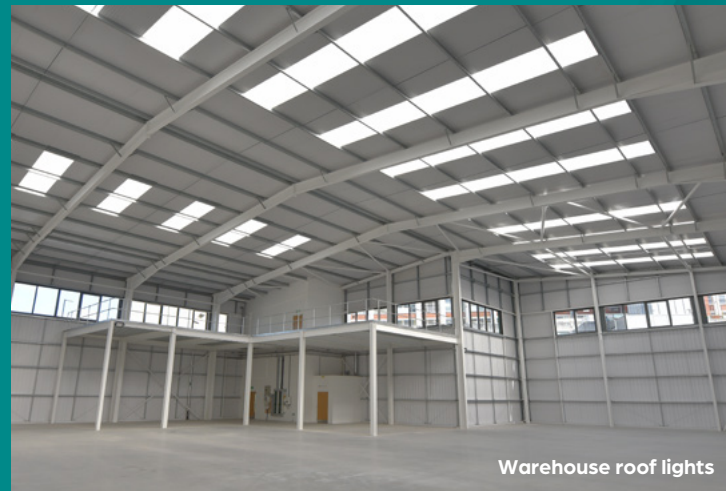
15% warehouse roof lights increasing natural lighting
